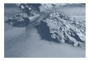
The basin contained 850 m³ (1 112 yd³) of mineral sludge, which was too harsh to use a conventional method, such as a centrifuge or a mobile press filter.
